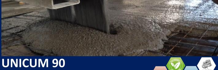
New generation superplasticizer additive, highly effective water reducer for high-quality precast concrete
